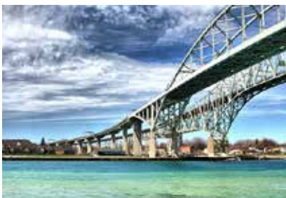
BLUE WATER BRIDGE
